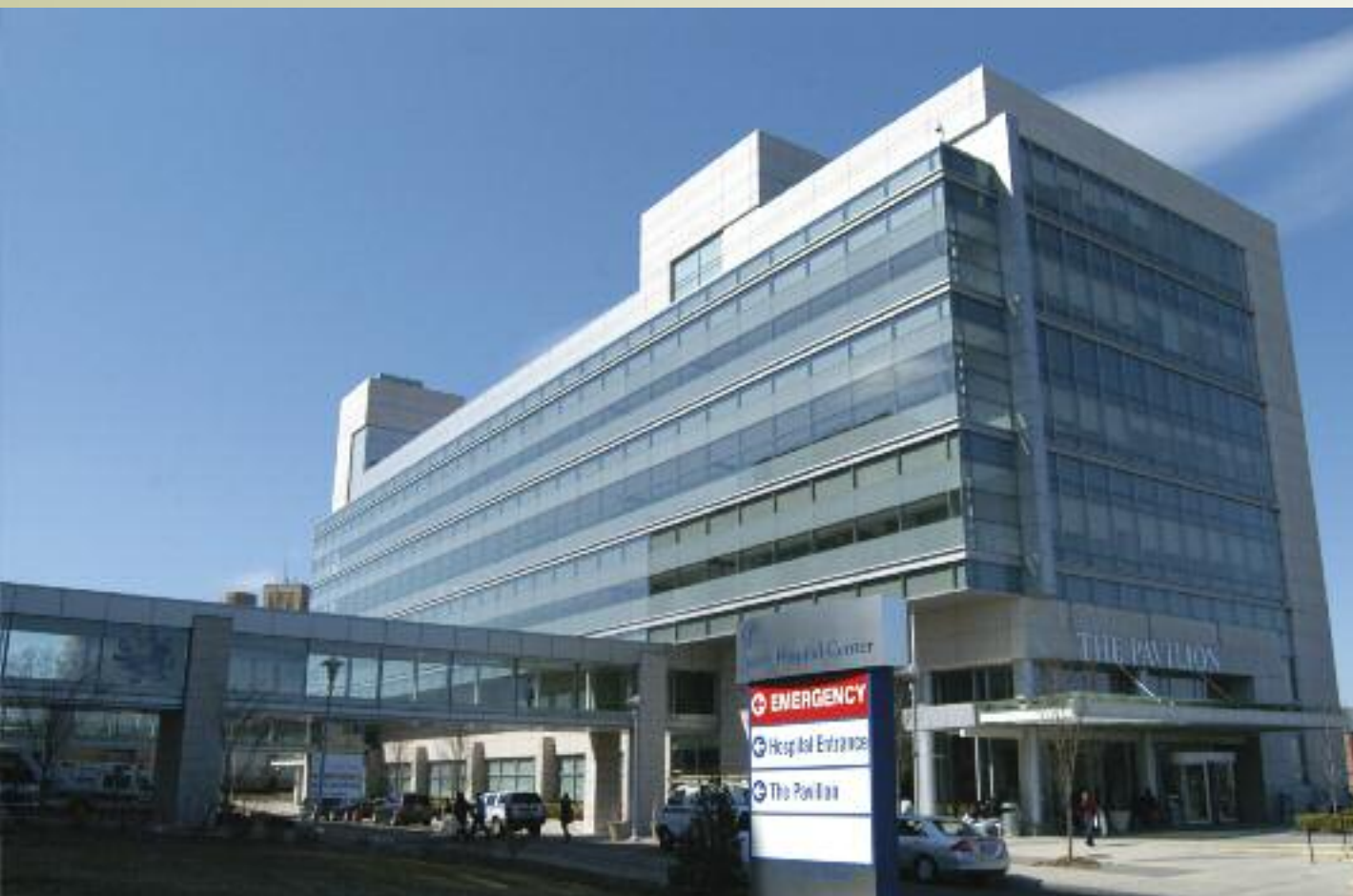
Photograph courtesy of Queens Hospital Center
